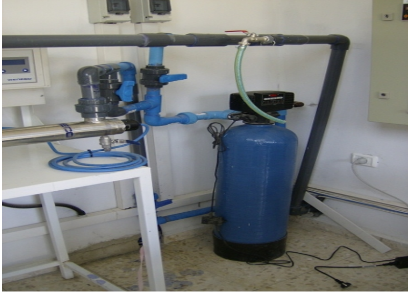
Photo 10: Multi-Media Granule Filter
